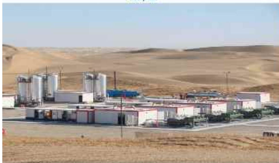
Wellgas recovery plant
