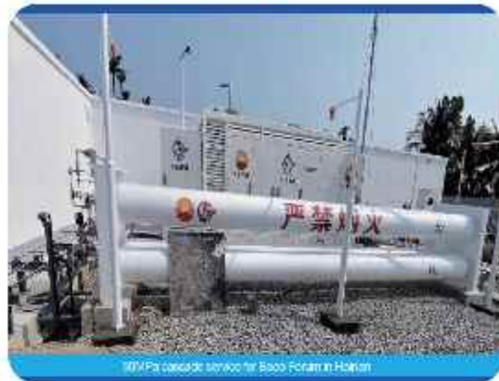
The National 863 Project - the first 70MPa hydrogen refueling station in China. ENRIC 70 MPa carbon wrapped cascade had successfully passed the test, which reaches the world's leading level in technology. It is also the first company in the world to adopt carbon fiber full-winding reinforcement technology in seamless steel cylinder, and this product has obtained multiple invention and patents.
